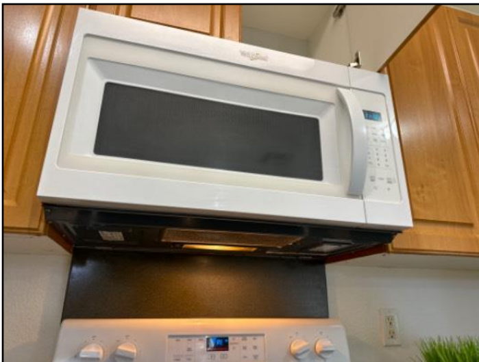
Microwave/Exhaust Fan functional
