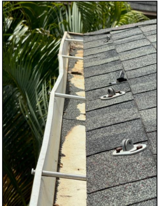
Damage/rock loss
